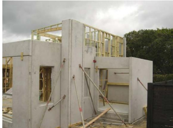
panel, usually at the 2-metre height. Four props for a two-storey panel; two at 2-metre and two at 4-metre height. Photo (at left) shows a Reid insert (TIM 16x75mm). A rod goes through the hole which is shown, prior to the panel being cast. The smaller end of the threaded inserts is set about 3mm below the panel surface and can be easily filled later.
