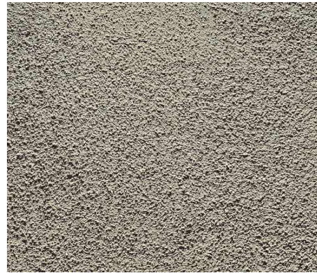
Sand Float is a popular, trowelled-on textured plaster finish available in several grades from light to heavy
